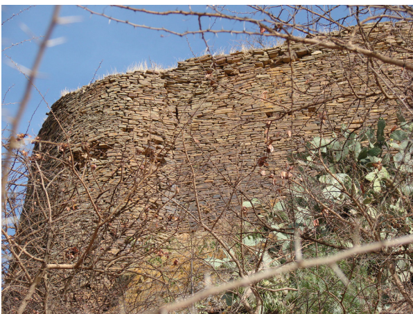
FIGURE 39. A detail of the dry stone masonry of the Fremona defensive walls and bastion. Photo by V.M. Fernández.
