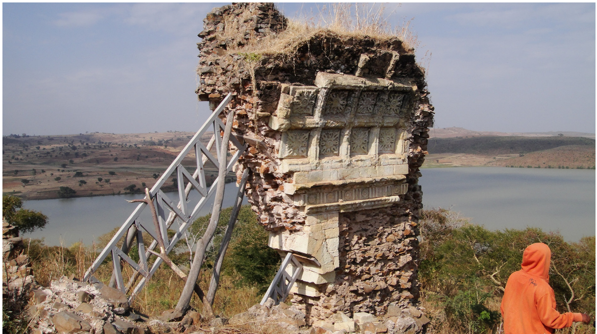
FIGURE 15. The apse of Gorgora Nova church after the protection scaffold was installed in 2009. Photo by V.M. Fernández.
